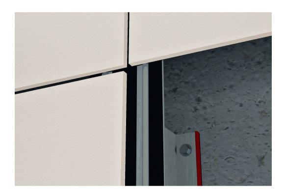
Close up of Lapitec slabs anchoring system to the walls
